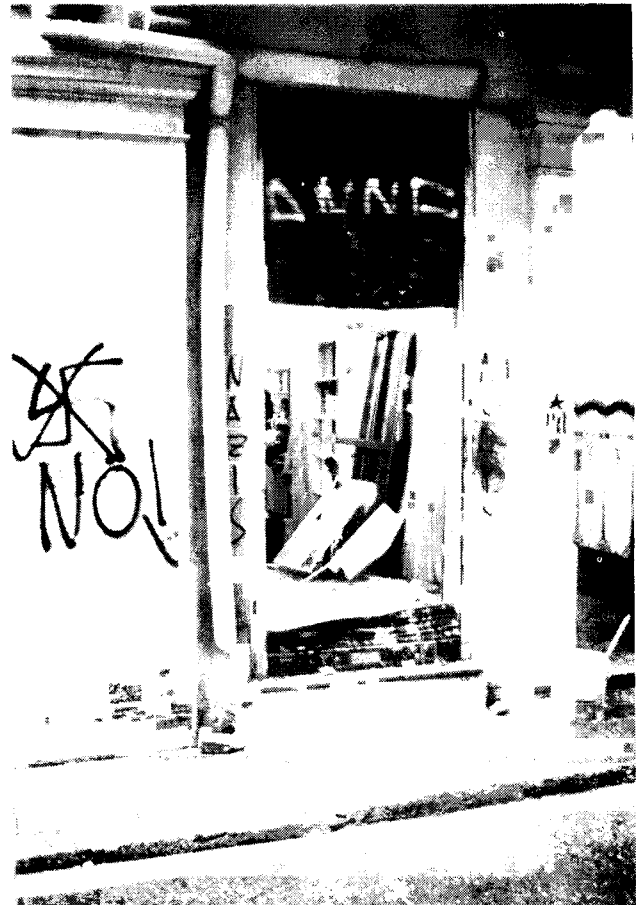
In their assault on the Europa bookstore on Barcelona’s Séneca street, the “anti-fascist” thugs broke through the roll-down steel covering that protected the front door. This photo was taken in the aftermath of the January 16 attack.
